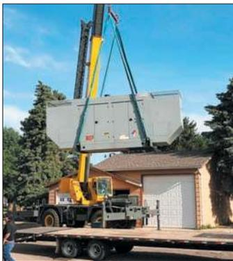
200KW generator lifted by Amert Construction crane.
