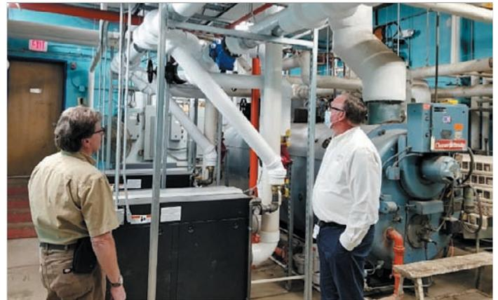
**Rick Barger of Barger Electric (left) and Chuck Johnson, CEO/Administrator of Bethel, viewing the recently installed modulating boiler and transport pipes system. The project was a major efficiency upgrade for the nursing home heating system and hot water needs.**
