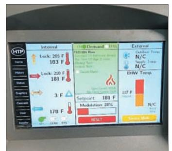
**Usage rate of 28% and generating heat temperature of 181 degrees that exceeds the state laundry water minimum temperature requirement.**
