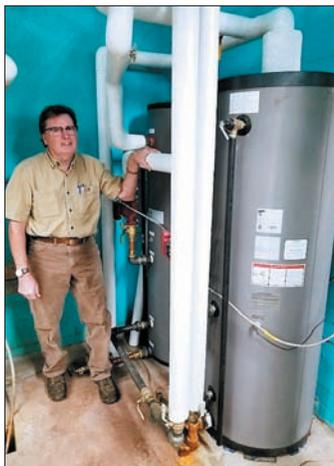
**Barger Electric Owner Rick Barger stands by the now incorporated laundry water heat system along with the building boiler. In the past there were two systems now collapsed for more energy efficiencies.**
